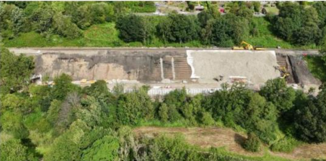
Hague Bar mid construction: Benching and rock fill placement ongoing, drainage being installed at the regrade toe.
