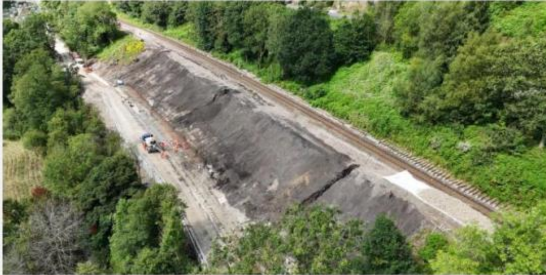
Hague Bar mid construction: contiguous piled wall installed and failed slope material removed ready for rockfill placement
