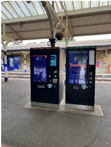
Figure 13: Two TVMs sheltered under a platform
