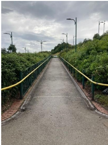
Figure 25: Ramp to Platform
