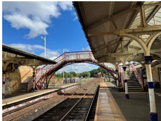
Figure 10: The foot bridge provided at Hexham to change platforms
