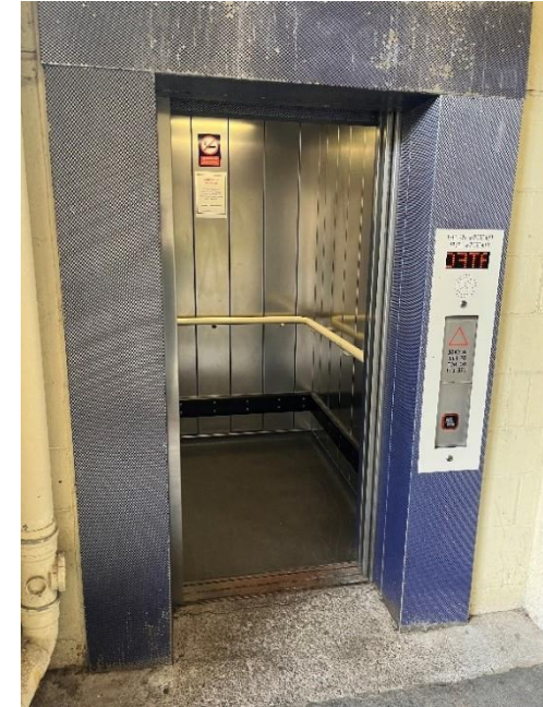
Figure 14: Lifts available to access the platform
