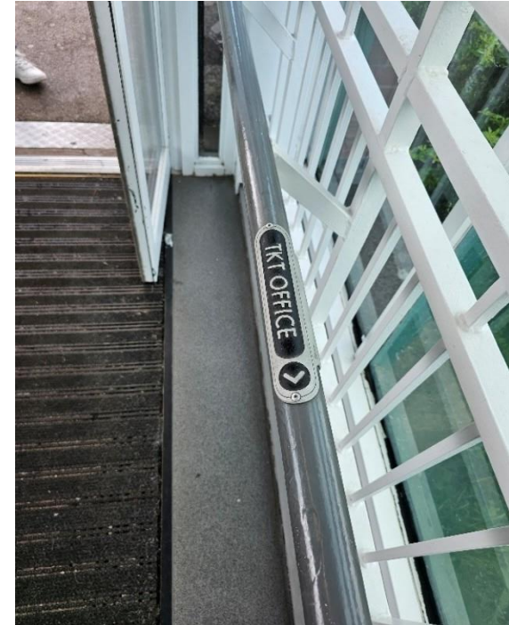
Figure 29: Braille signage on platform towards the TOs
