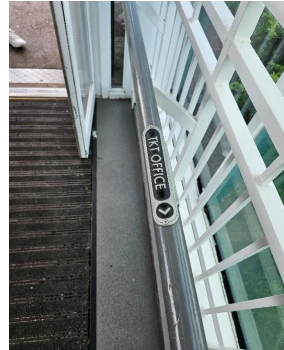
Figure 29: Braille signage on platform towards the TOs
