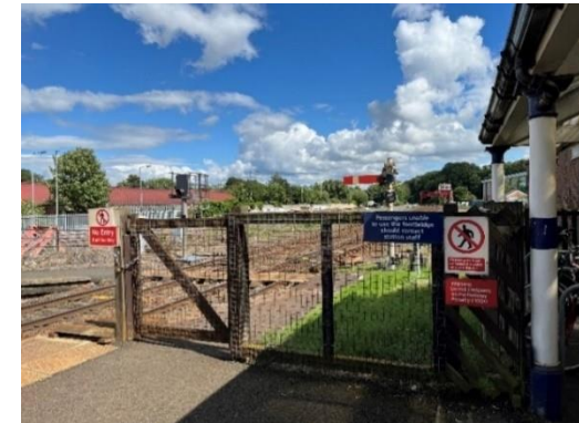
Figure 12: Signage requesting those passengers who are unable to utilise the footbridge to contact staff
